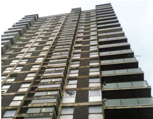
Original 1960s facade
