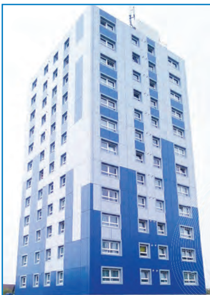
NOVEMBER 2017 – RECLAD COMPLETE TO MEET 2019 STANDARDS
