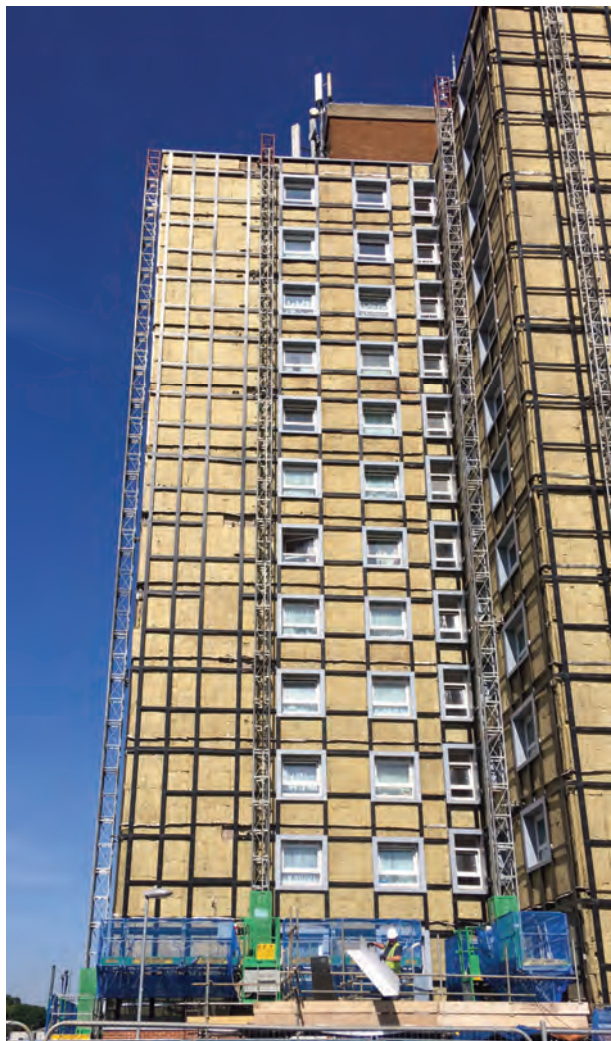
The combustible cladding was removed within 10 days.
