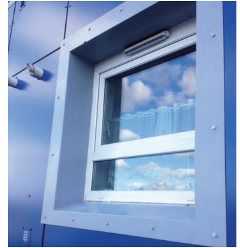
Window and POD clean after new cladding installed.
