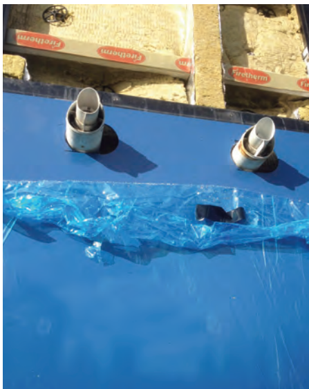
Non combustible Flue panel installed.
