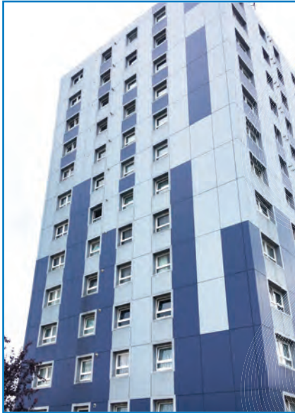
Clements Court 23rd June LBH become aware of fire hazard.
