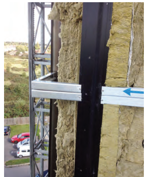
Support structure replaced where missing.
