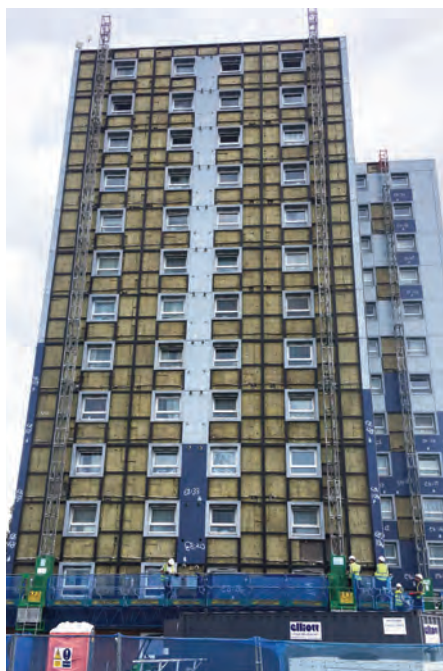
Combustible panel removal uncovers the insulation and firebreaks.
