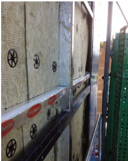
Closeup of new firebreak & insulation.
