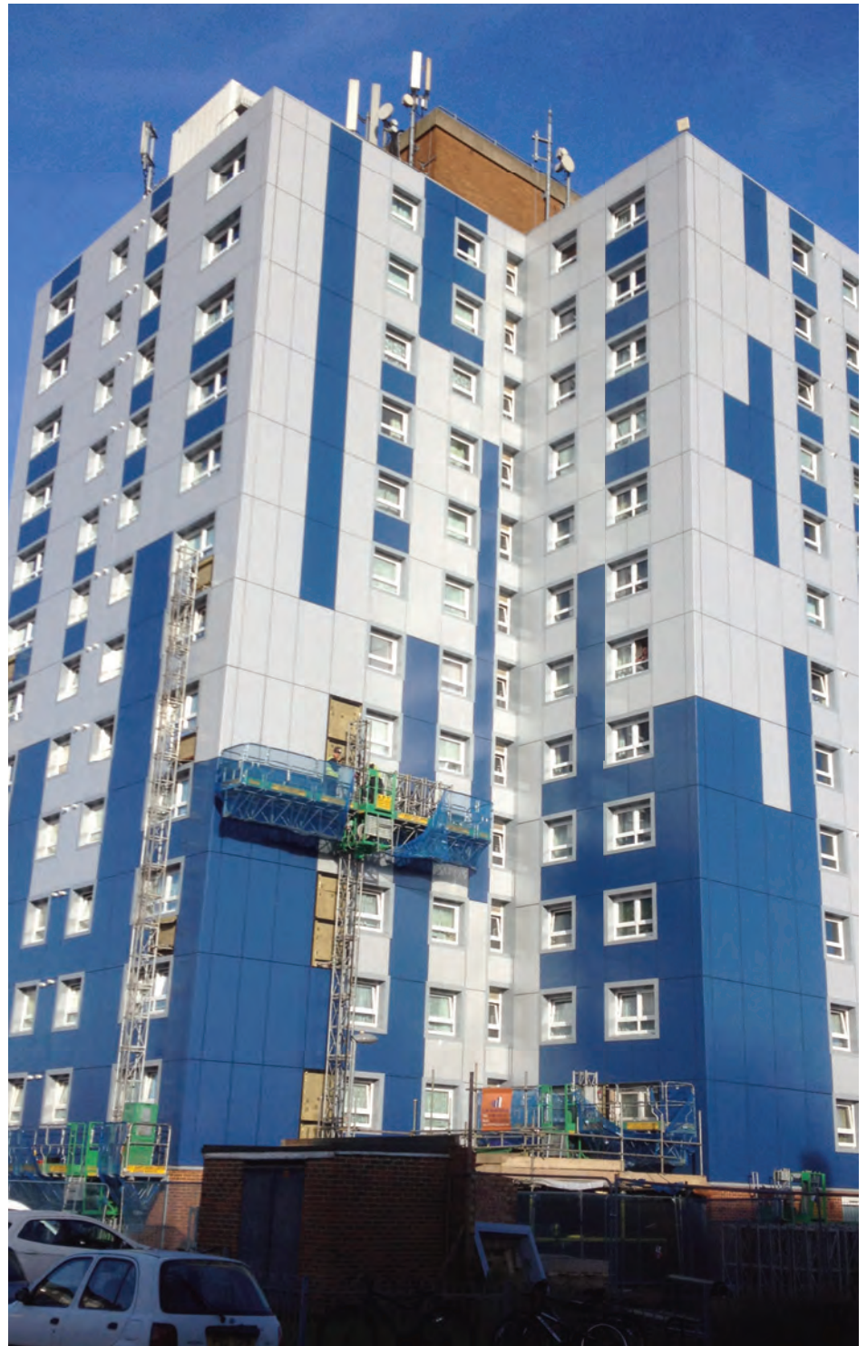
Access under removal.
