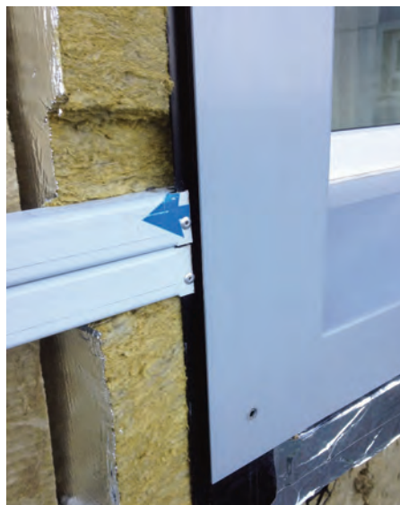
Support structure replaced where missing.
