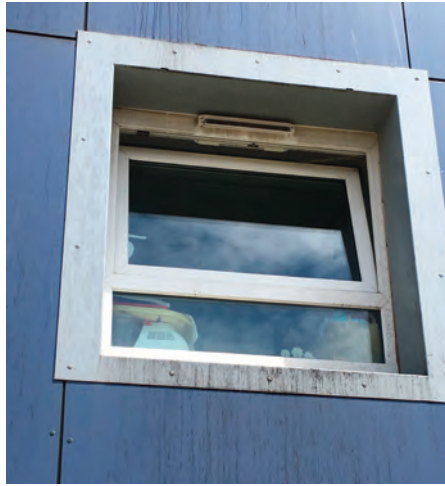
Window and POD before clean and cladding replacement.
