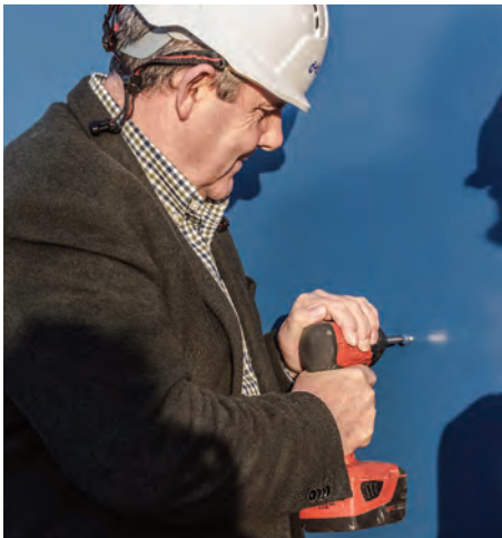
Cllr Steve Curran (Council Leader) securing the last non-combustible panel.
