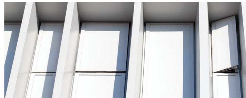
The final solution met the architectural intent that "Veil" should have no visible windows whilst meeting the performance requirement of transmittance of light internally.
